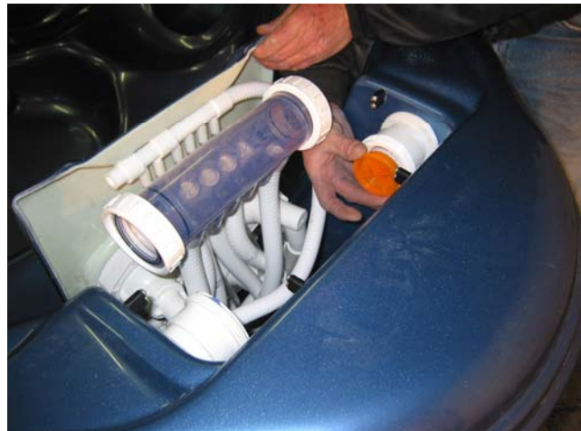
(Figure R) Location of Jet Zone Divider
