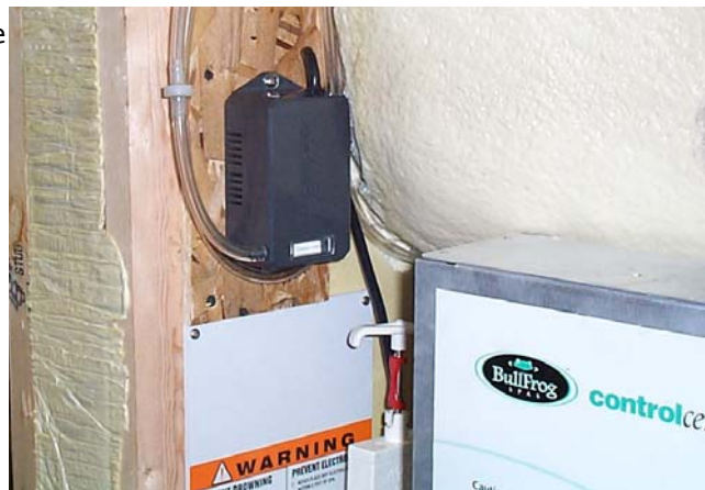
(Figure V) Ozone Sterilizer Location
